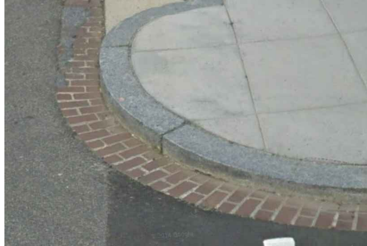
3 DDOT GRANITE CURB AND BRICK GUTTER
