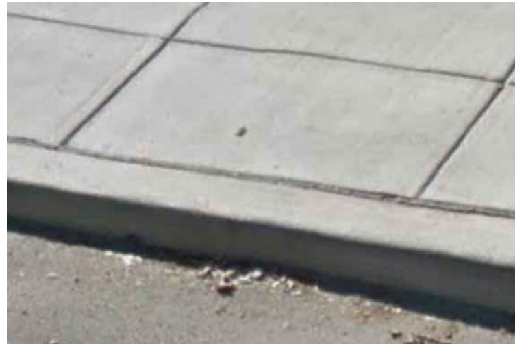
2 DDOT CONCRETE CURB
